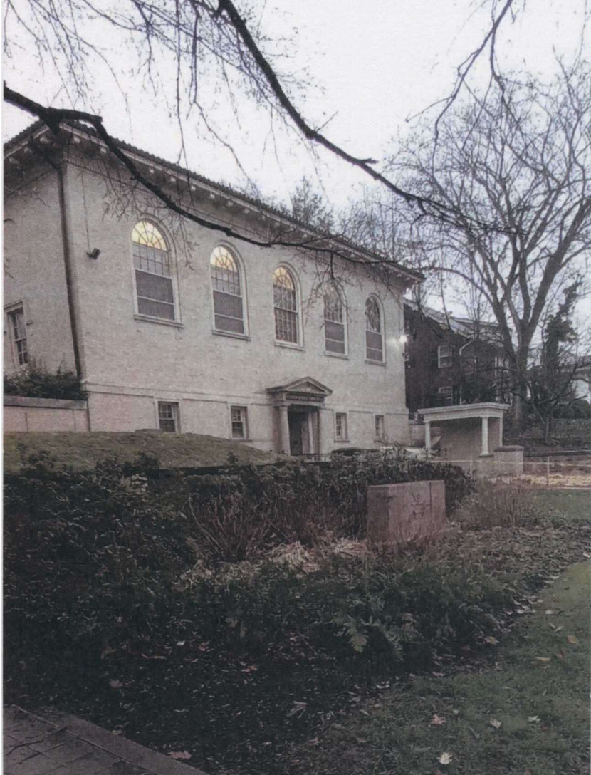
The completed brick enclosure on the north side of the library awaiting the arrival of the new pick-up lockers, November, 2022.
